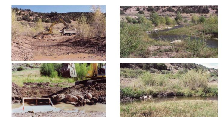
Pictures of the Hall project during construction are shown on the left (new channel reconstruction, and fish structure next to a rock barb), and photographs on the right show the same place after about 2.5 years.
