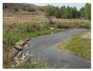
Photographs above are taken about 2.5 years after the project and illustrate rock vanes deflecting flow away from the toe of the bank, barbs that move the flow toward the center of the channel, and re-established vegetation.
