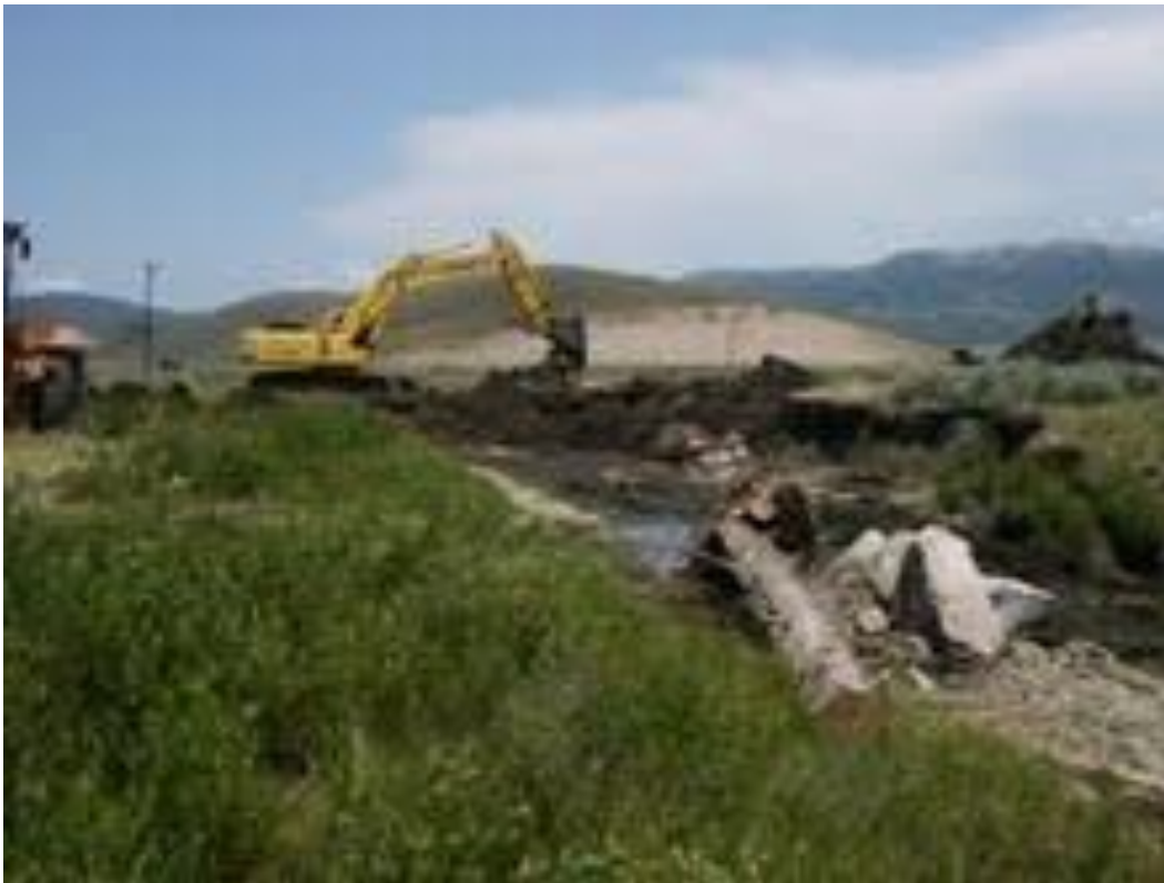
FIGURE 2. FIGURE 2. STRAWBERRY RIVER (SAME REACH) DURING RESTORATION ACTIVITIES IN 2002 INCLUDED INSTALLING STREAMBANK STABILIZING STRUCTURES.
