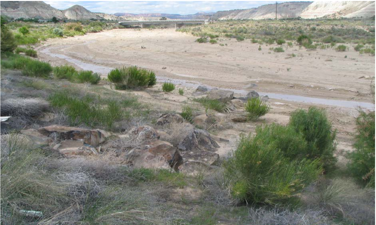
Additional view of rock barbs and sloping on Paria River Restoration Demonstration Project, looking north toward Highway 12 at Cannonville Bridge. (June 2009)
