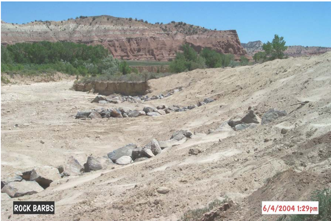
Additional view of sloping and rock barbs on Paria River Restoration Demonstration Project (June 2004)
