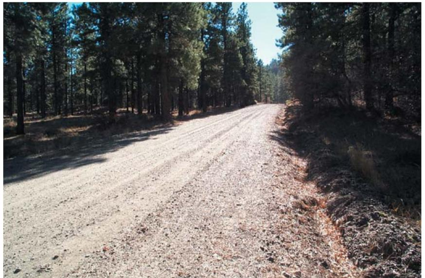
*This forest road is located well away from water. Its gravel surface promotes drainage and lessens erosion. The road is crowned, so water drains away to both sides.*
