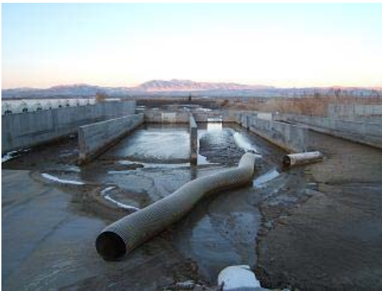
Figure 8: Solid and liquid bunkers. Previously Wash water and runoff would run into the Cub River. (Richmond Utah #14)
