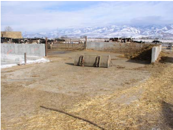
Figure 2: Concrete waste storage structure (Lewiston, Utah #1)
