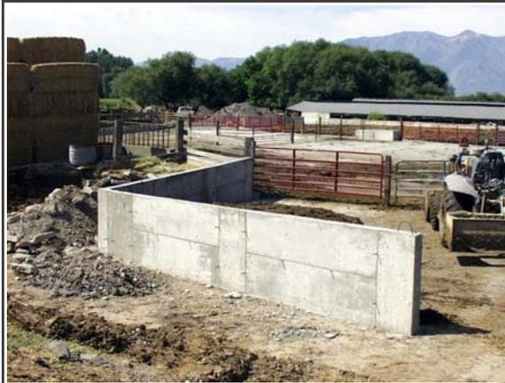
Figure 4: Manure storage bunker
