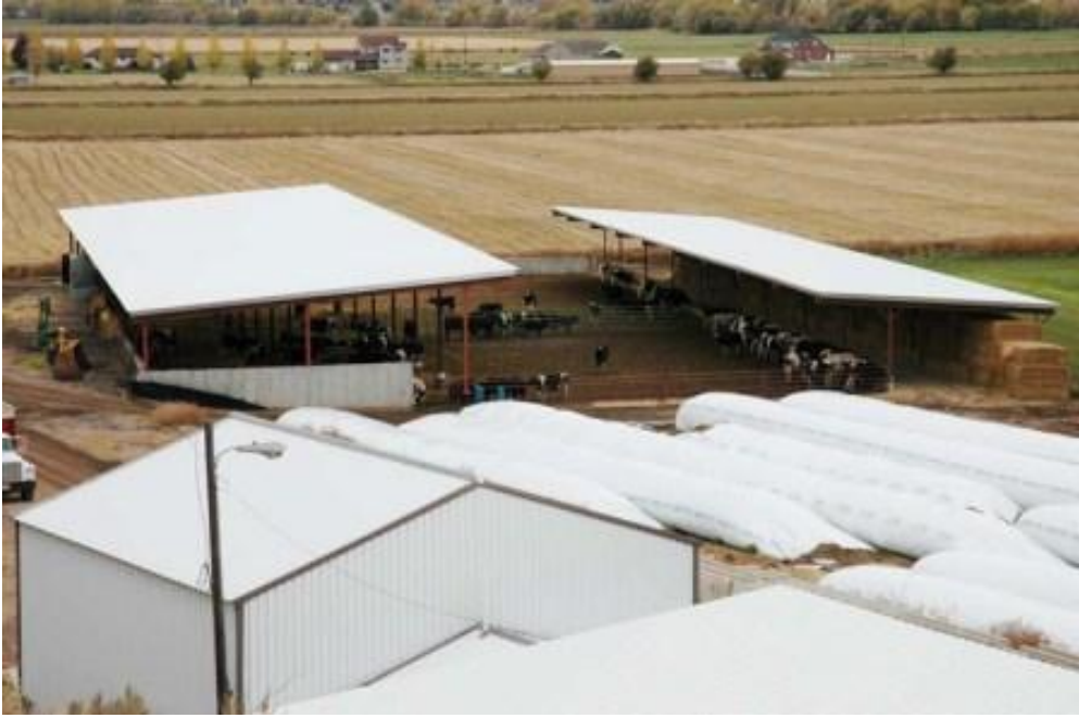
Far view of completed project area
